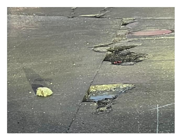
A pothole is a depression in a road surface, usually asphalt pavement where traffic has removed broken pieces of pavement. It is usually the result of water in the underlying soil structure and traffic passing over the affected area.
