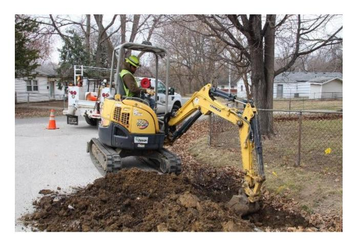
**ALTON** – Ameren Illinois customers in and around Alton and Godfrey will see energy at work throughout the spring and well into the fall as crews replace steel pipeline and natural gas services with modern, corrosion-resistant polyethylene material.
