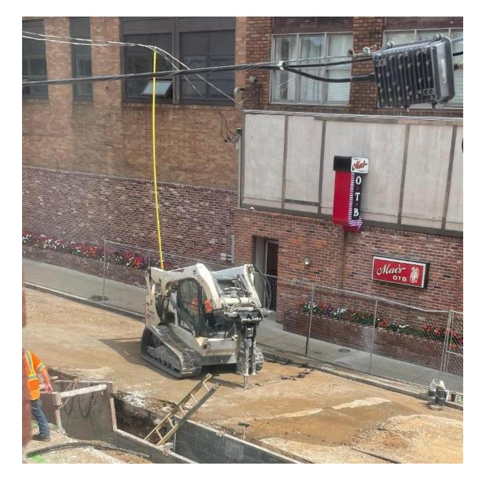
Illinois American Water's recent work has been to separate the Alton combined sewer system and install new sanitary sewers. Additional work is still needed in other areas and more information on that is below.
