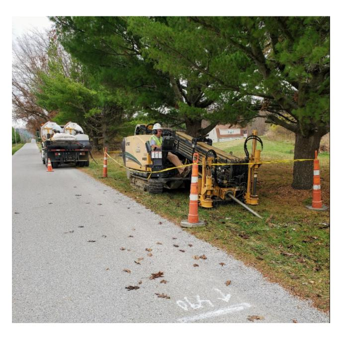
**PONTOON BEACH/ALTON/GODFREY** - Ameren Illinois customers in and around Madison County will see energy at work firsthand throughout the spring and well into the fall as crews replace vintage steel pipeline and natural gas services with modern, corrosion-resistant polyethylene material.
