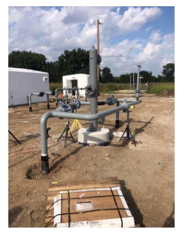
ALTON – Ameren Illinois is investing \$1.3 million to update the natural gas system in Alton. Last month the company began the installation of new equipment at a local gate station – the point where natural gas is received from interstate pipelines and transferred into the local distribution system for safe delivery to customer homes and businesses.
