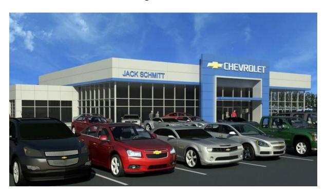
The 33,000-square-foot dealership will be a new prototype Chevy dealership on an 11-acre site. It will be a pre-engineered metal building frame with some masonry,
