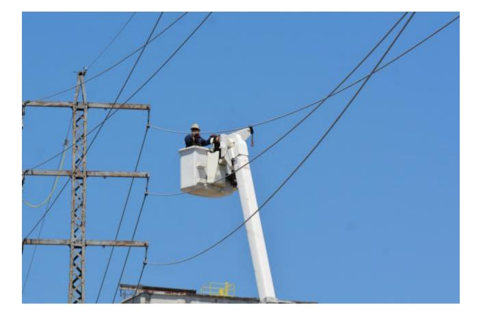
ALTON - J.F. Electric was visible at work high in the air late last week after lightning struck a static line on top of a pole near Argosy in Downtown Alton.
