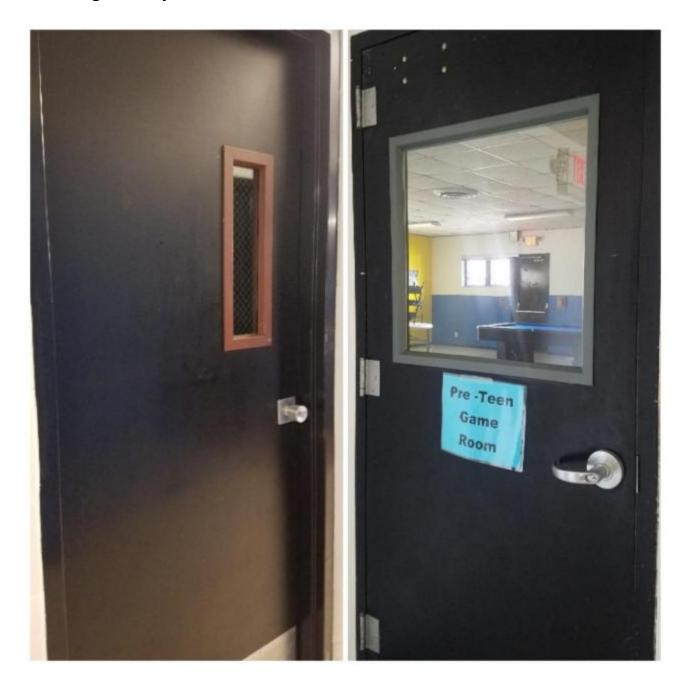
The project consisted of nineteen 24" x 24" tempered safety glass light kits for program doors, 200 square feet of laminate flooring for two personnel offices, 500 linear feet of wall base and a 3-person crew with 142 hours of time dedicated to the facility upgrades.
