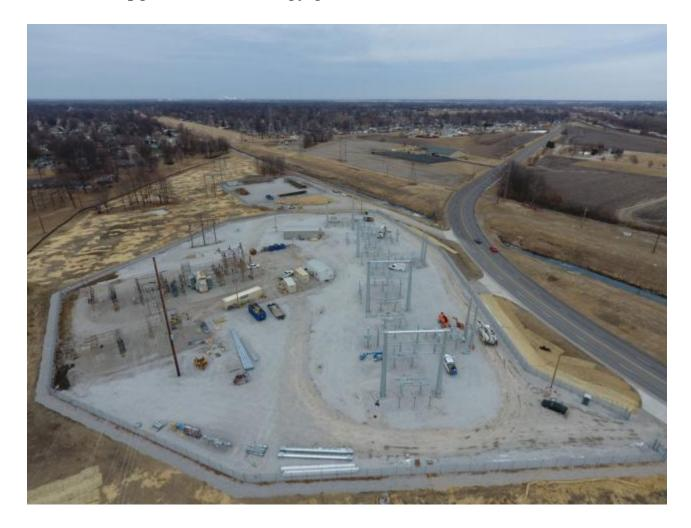
A transmission substation is much larger in size than a neighborhood distribution substation. It steps down high voltage it receives to a much lower voltage that can be transferred to a distribution substation. The distribution substation then steps down the voltage even further for delivery to small transformers, which starts the process of lowering the voltage for delivery of power to a customer's home or business.
